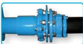
1. Bolt one flange of the HAWLE-VARIO with the counter flange (at the pipeline).
