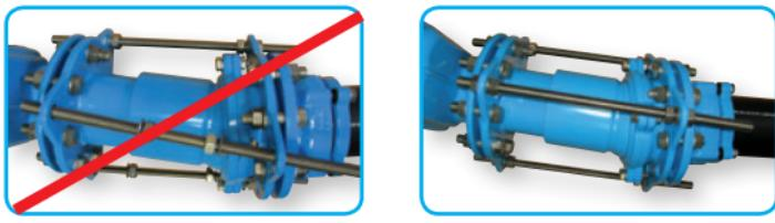
5. Tighten all nuts free from tension (max. 30 Nm).
